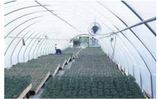
Greenhouse built on slope, must keep plants level.
